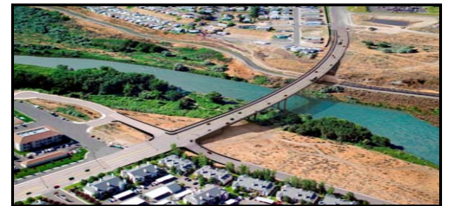
The city continued its pre-construction work on the Duportail bridge, which will span the Yakima River.
